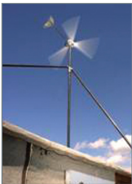
1.5 kW wind turbine
